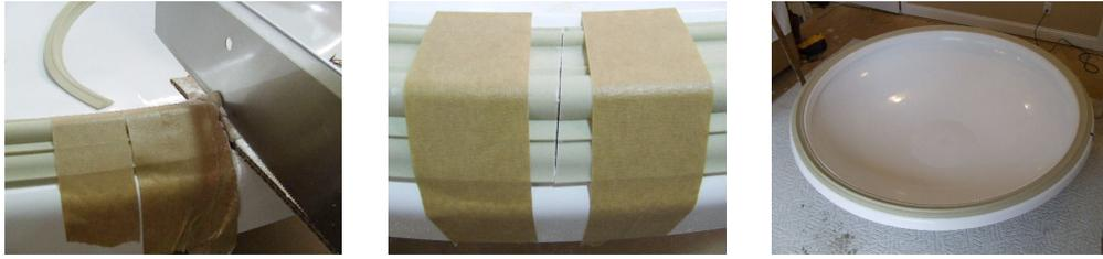
The splices are made on the dome prior to screwing down. When cutting the miter and removing the excess millwork. Place a piece of cardboard under the decorative trim. This protects the cove ring from damage.
